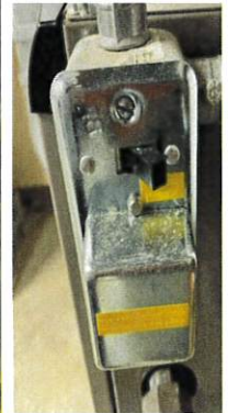
Shut off valve is located on the side of the unit (or the front for unit 2). Just flip the switch!
